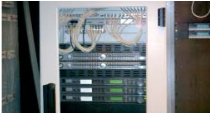
Three MA NSPs incl. backup are providing the necessary processing speed for the 4,000 control channels
