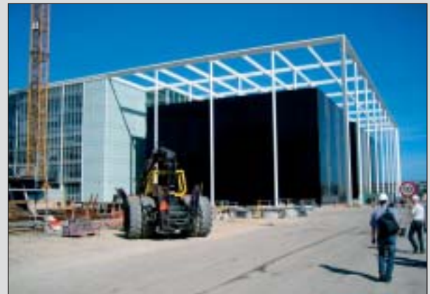
DR Byen's new home under construction
